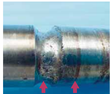
Damage due to overload and seepage
